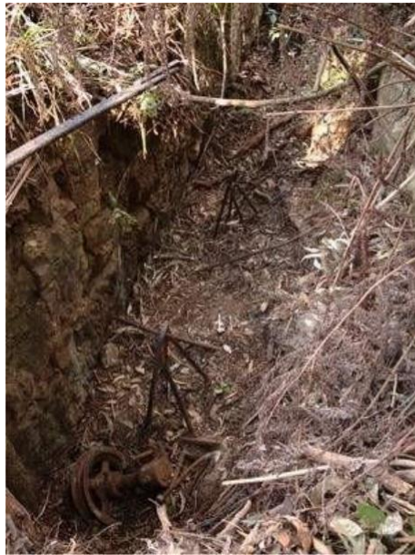
Figure 4.24 View down into the tension pit, showing three surviving counterweight cradles and remains of a chain roller in the foreground (looking south). (Photo: P1070495)
